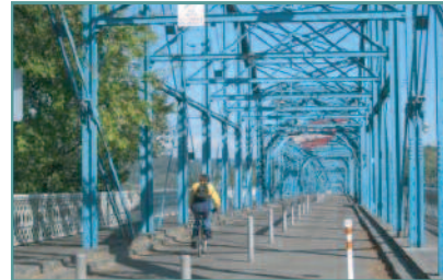
Walnut Street Bridge renovated for pedestrian use between South Shore and North Shore developments
