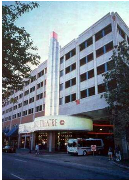
An electric bus enters Shuttlepark North. The CARTA terminal provides upper-level parking for hotel guests and downtown visitors. The Bijou Theater cineplex on the ground floor extends mixed-use development and defrays shuttle costs.
